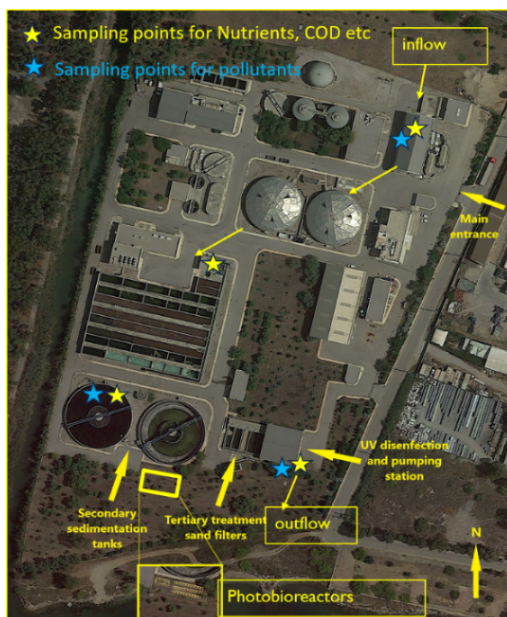
Fig. 1. The microalgae bioreactors system at Thrasio WWTP.
