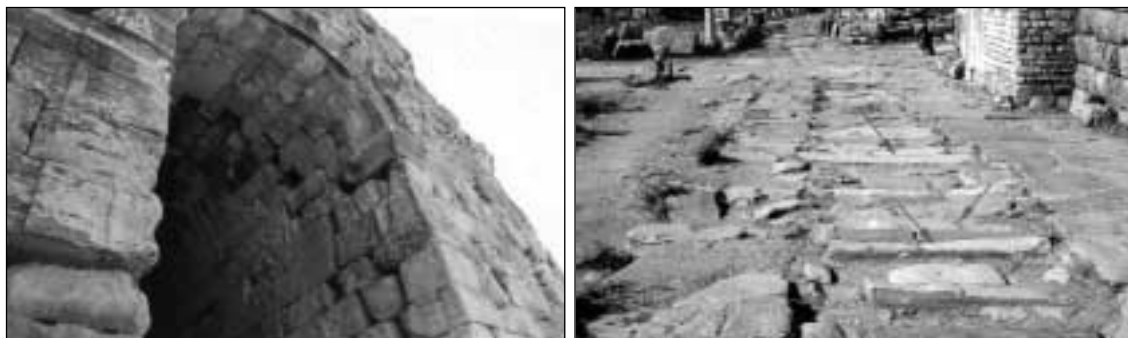
Fig. 5. (a) Northern entrance to the theatre in Miletus. Note that walls are dilated. (b) A reconstructed street in Ephesus. Note that columns were used (red arrows) and they were not eroded as much as other block stones (blue arrows).
