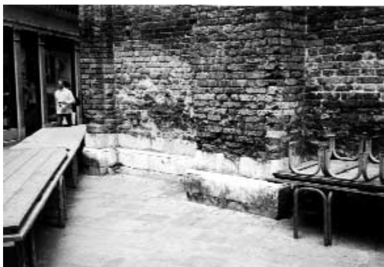
Fig. 4. Mobile footbridges near Frari church to make possible walking on flooded streets during acqua alta.
