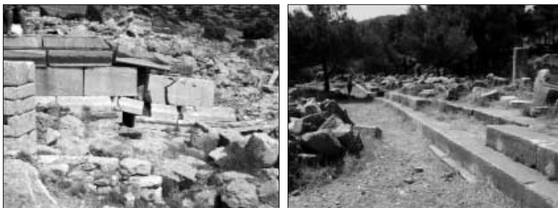
Fig. 6. (a) Offset in the Temple of Aphrodite Euploia in Cnidus. The south side was downthrown about 35 cm. (b) Stoa in Priene, where the northwestern side was downthrown about 50 cm (red arrow) along a NE-SW-trending zone.
