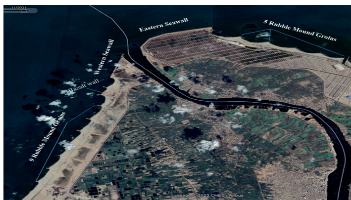
Figure 16. The current protective structures along the Rosetta Promontory.
