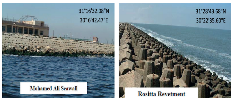
Figure 6. Examples of the implemented hard structures as a protection adaptation option to SLR (Iskander 2010).
