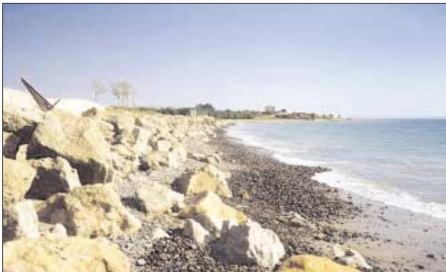
Fig. 3. The beach of Montroig (Tarragona, Spain), eroding as a result of (nearly complete) up-drift longshore transport reduction.
