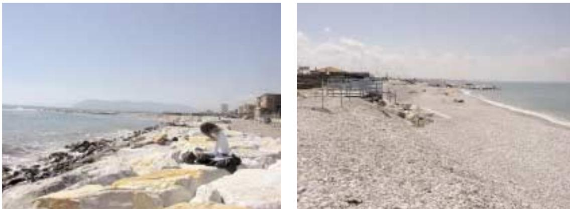
Figures 1 and 2. Tuscany coastal protection (groins and dykes) made with marble blocs and gravel.
